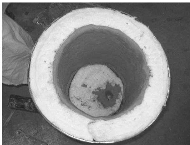
Figure VI-6: Hotface sidewall installed in the furnace
