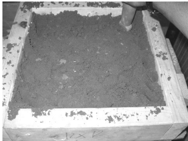
Figure III-13: Beginning to ram
