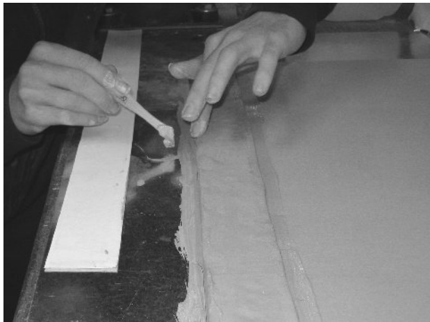
Figure VI-5: Blending floor support strip into hotface sidewall
